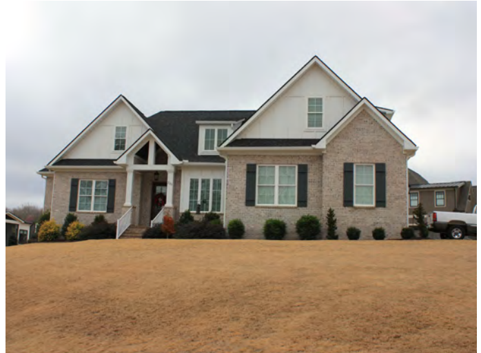
Single family homes make up over 70% of the existing housing stock in the City of Fountain Inn.
